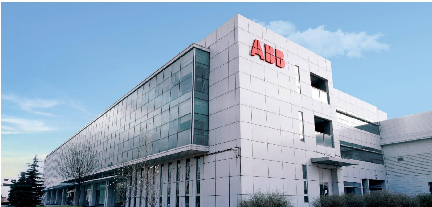
ABB High Voltage Switchgear Co., Ltd., Beijing, China
